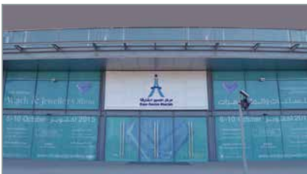
Al mamzar entrance Vinyl Glass Panels: 7 X 2.5 M
